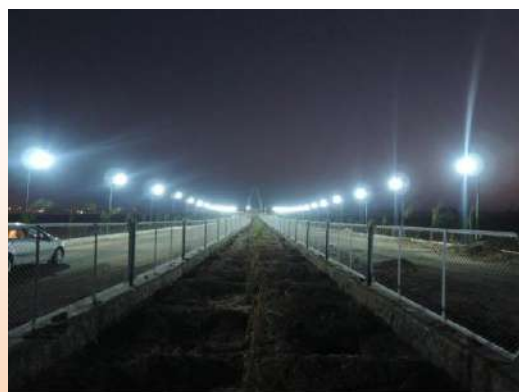
Solar Lights in the Campus
