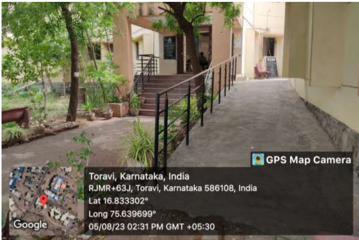
Ramp – Education Building
