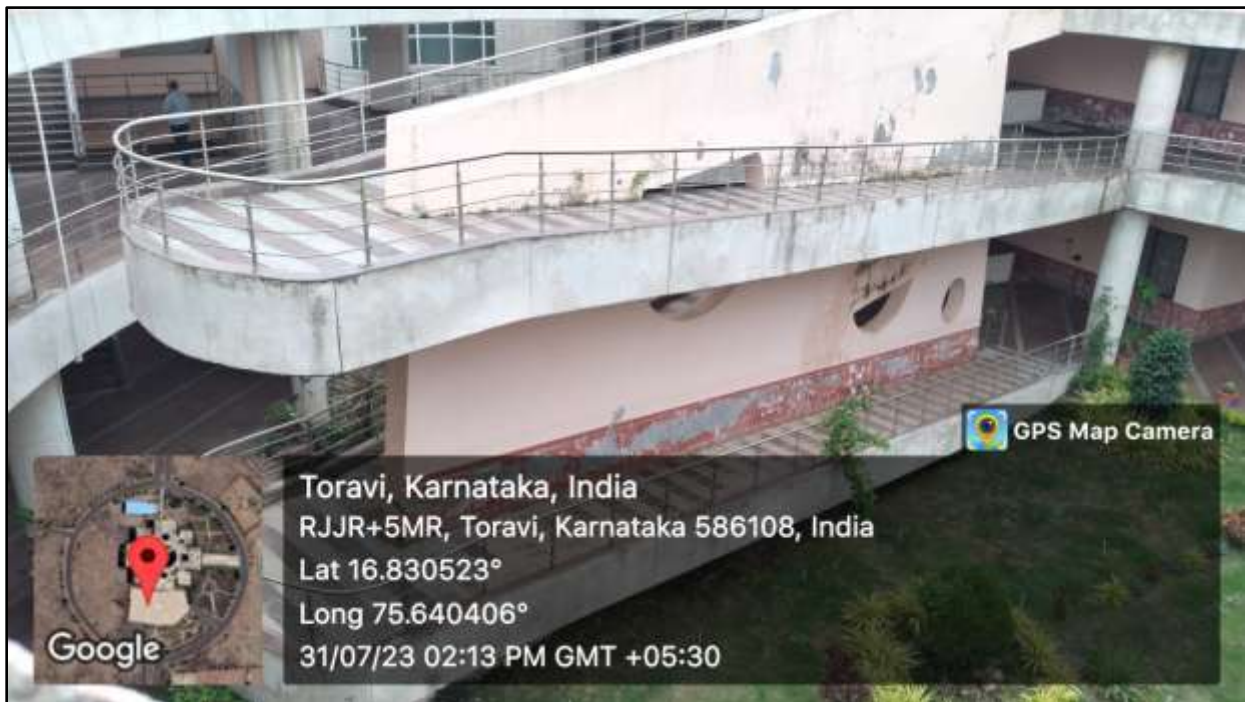
Ramps – Administrative Building
