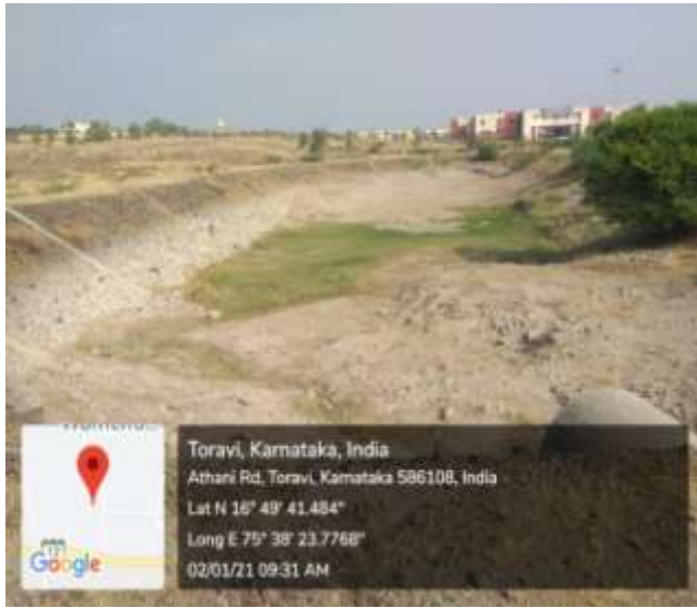
a) Runoff Storage Ponds
