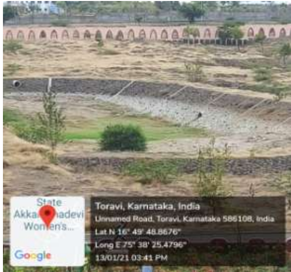
a) Runoff Storage Ponds
