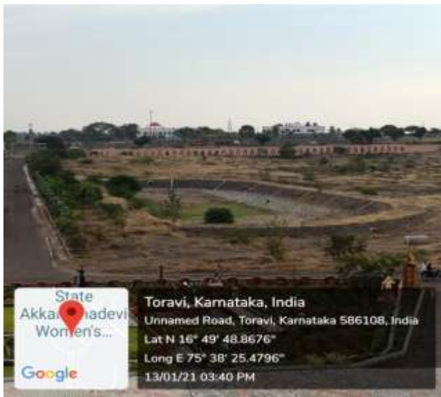
c) Rainwater Storage Structures
