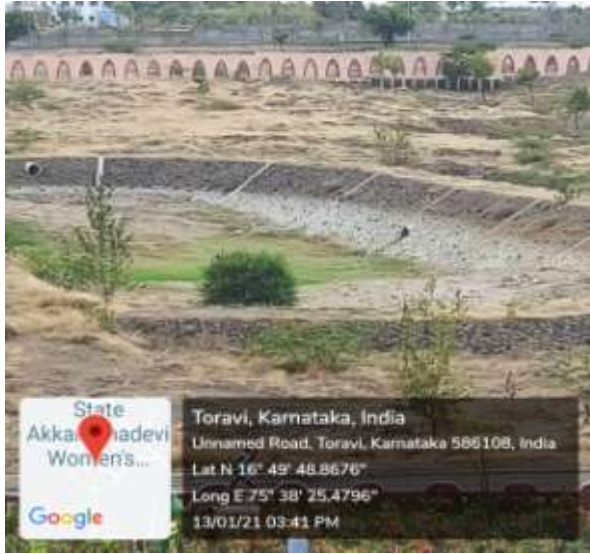
a) Runoff Storage Ponds
