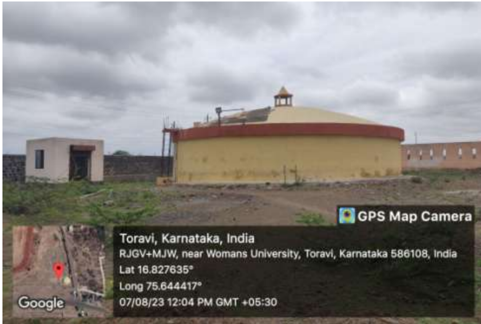
Water Storage Tank 1: ( Storage Capacity- 12 Lakh Liters)
