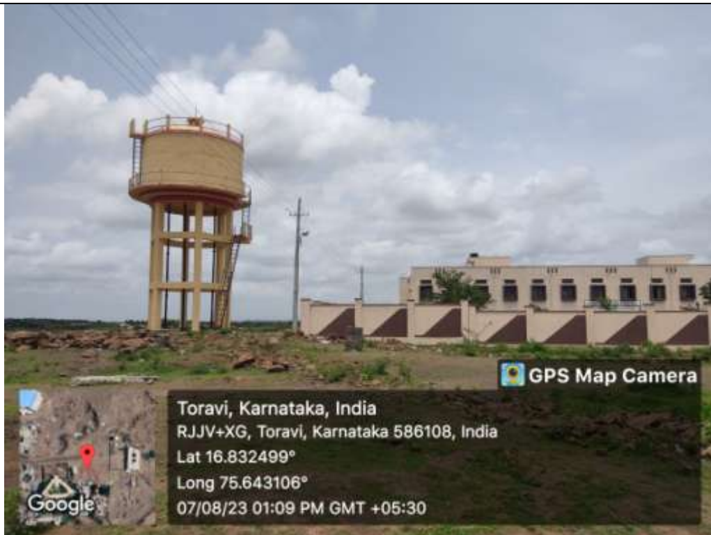
Water Storage Tank 1: ( Storage Capacity- 2 Lakh Liters)
