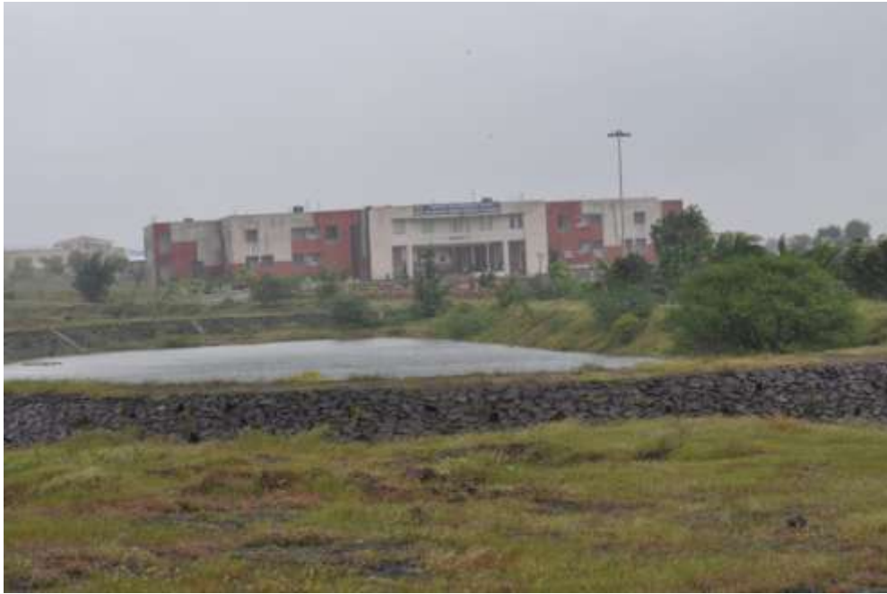
Pond constructed in front of Administrative Block
