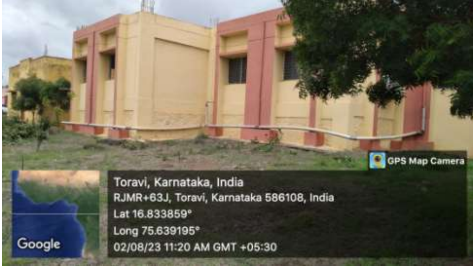
Rain Water Harvesting System
