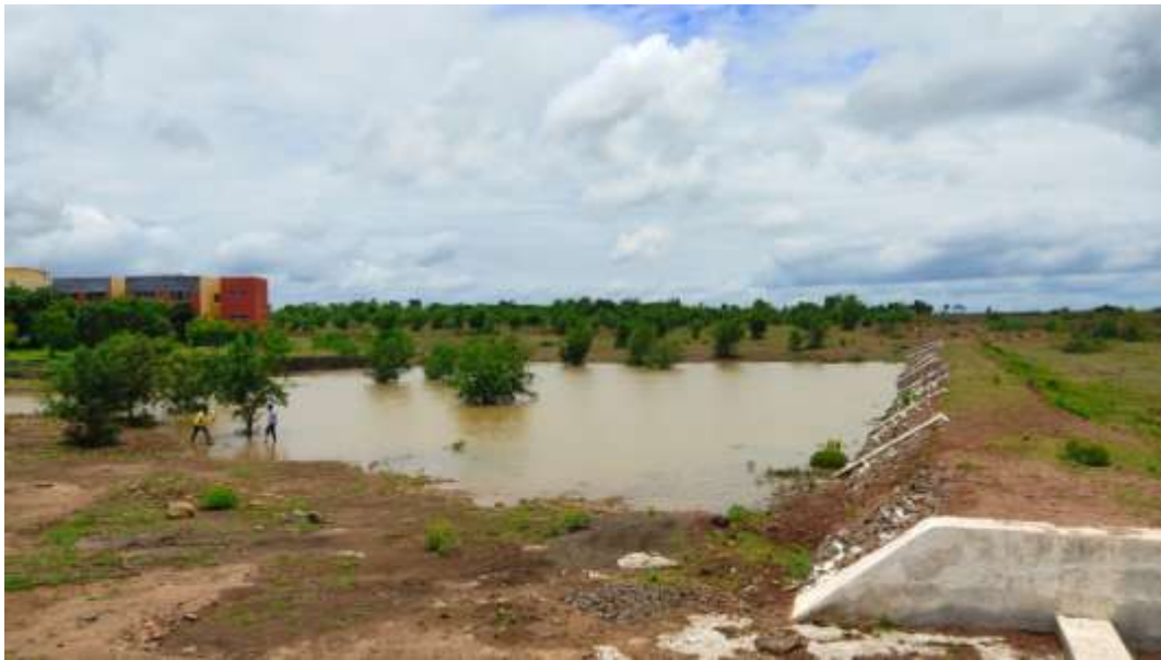
Bund constructed in front of social science block
