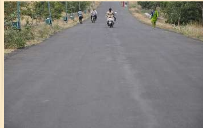
Development of internal roads
