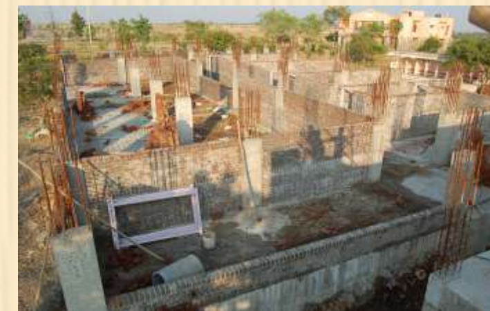
Construction of Library Building First Floor
