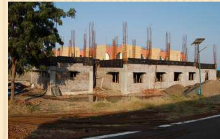
Building construction of Dept. of Electronics
