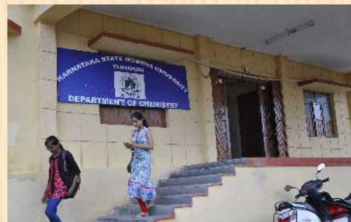
Chemistry Dept. Building Renovation
