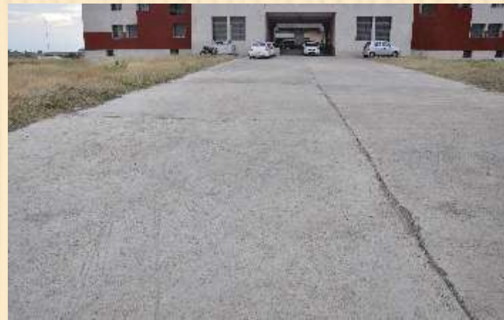
Construction of CC Road
