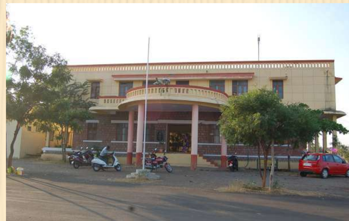
Renovation of MLISC and JMC Building
