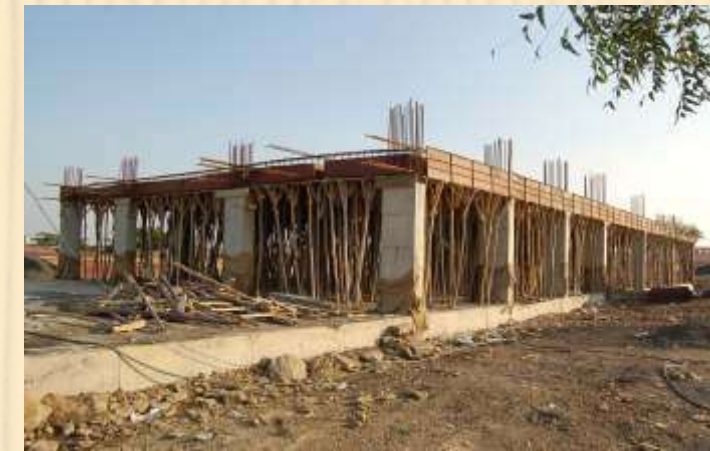
Building construction of Dept. of Physical Education
