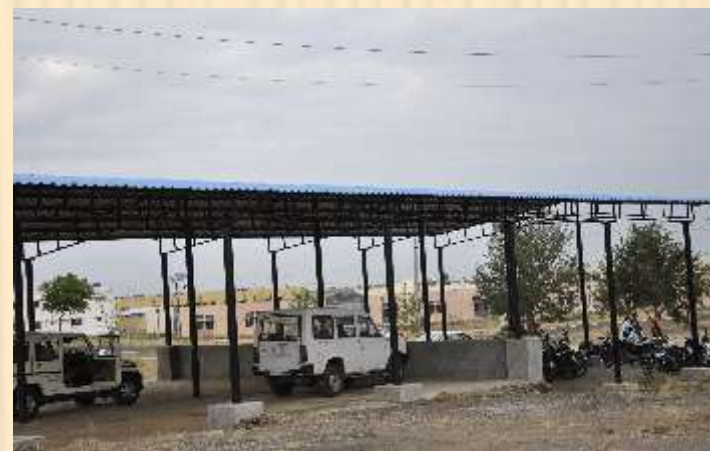
Car and Bike Parking Shed
