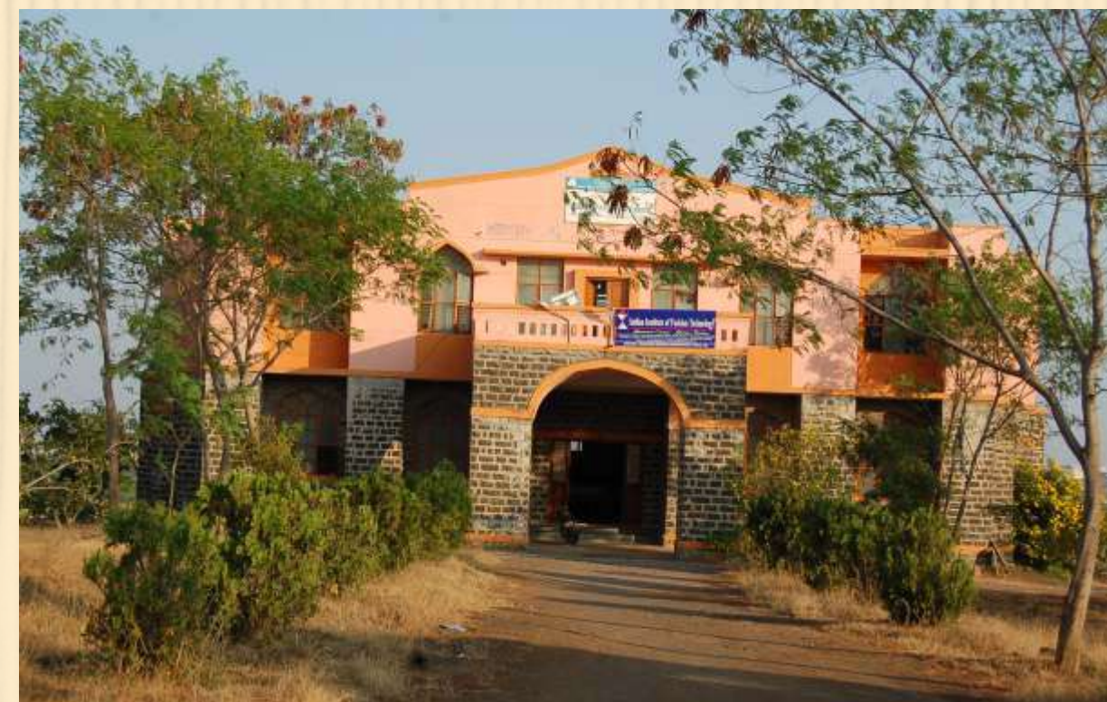
Renovation of old ADM Building
