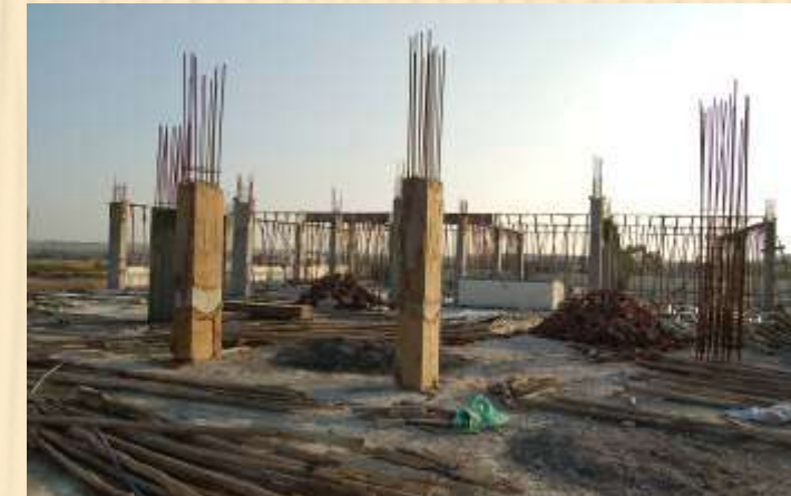
Construction of Library Ground Floor
