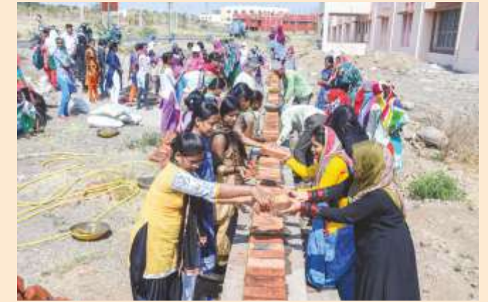
NSS Students constructing a compound wall
